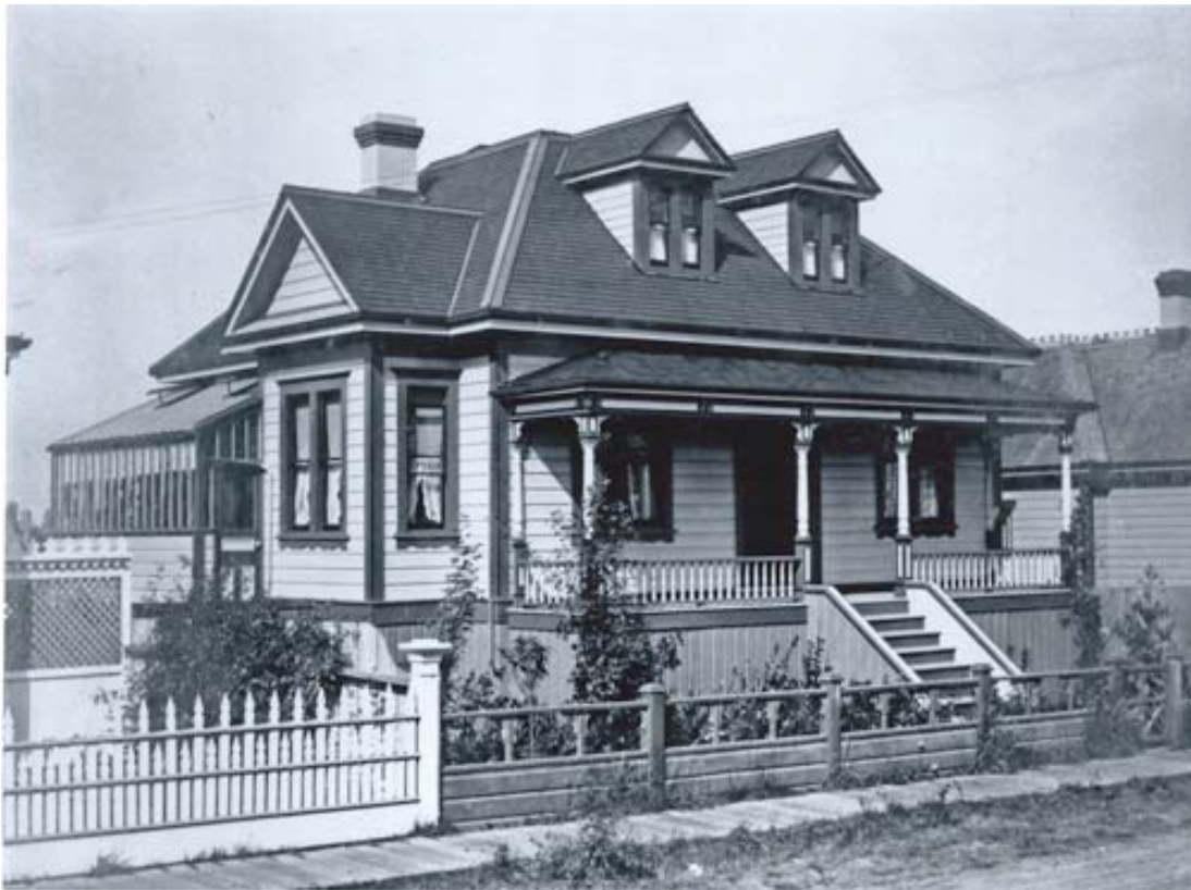
Circa 1901 photo of house built by John Lewis at 58 Government Street, Victoria, Canada (Photo by John Lewis)
